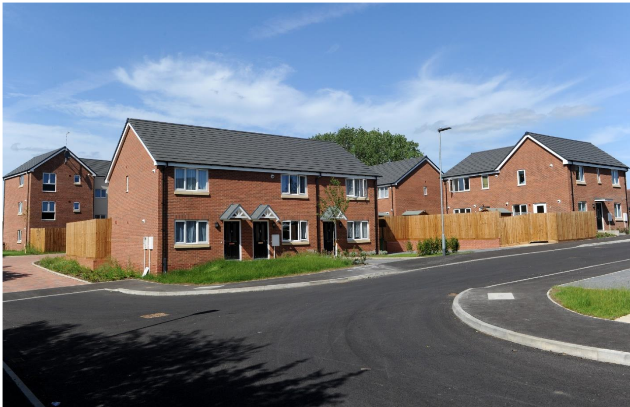
Figure 1: Photo of completed homes at Belle Vue
