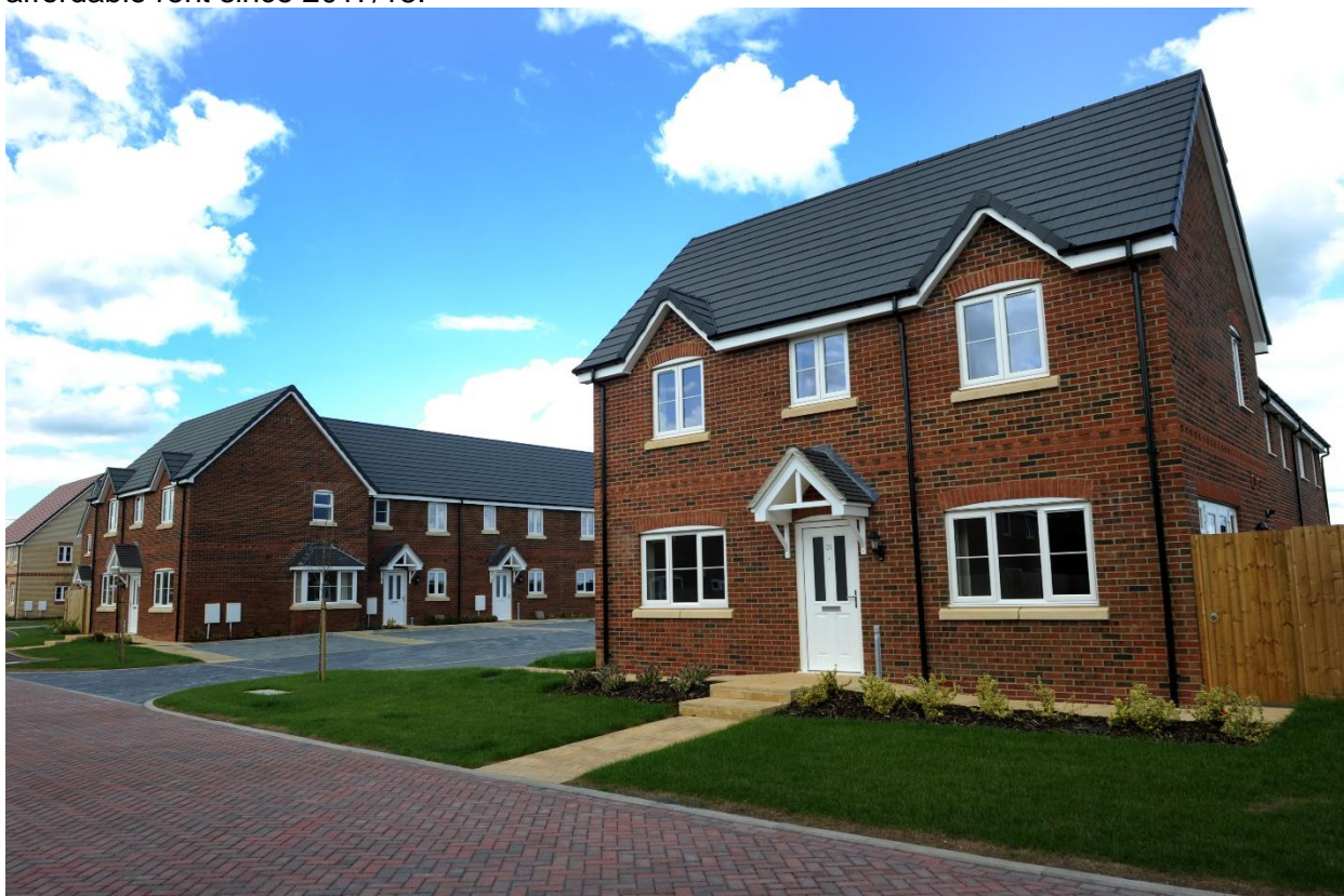
Figure 2: Photo of completed homes at Crowland Road
